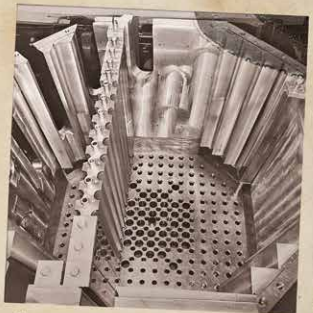
Fragment of the reactor core with aligned core matrix and reflector blocks
